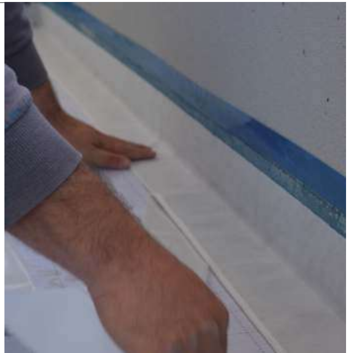
BRW PFN SHEET MEMBRANE | FLOOR WALL JUNCTION TERMINATION
